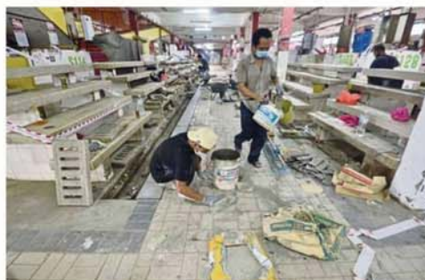
Long overdue renovations are currently taking place at the market.
